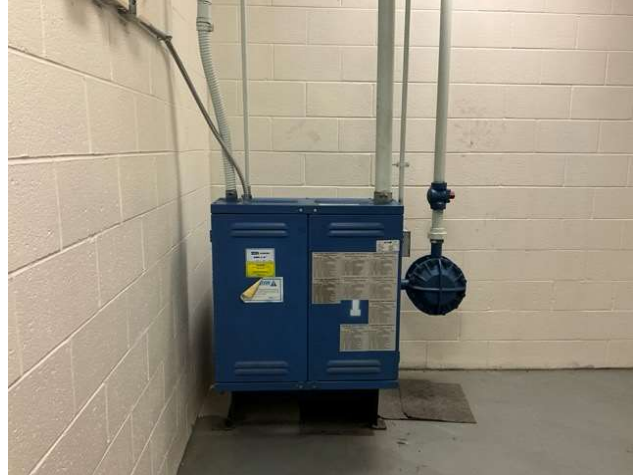
26 - ELEVATOR CAB PANEL
