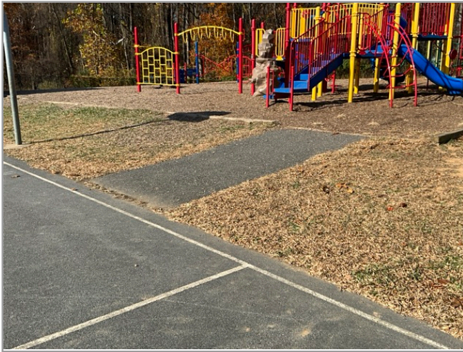
ACCESSIBLE ROUTE TO PLAYGROUND
